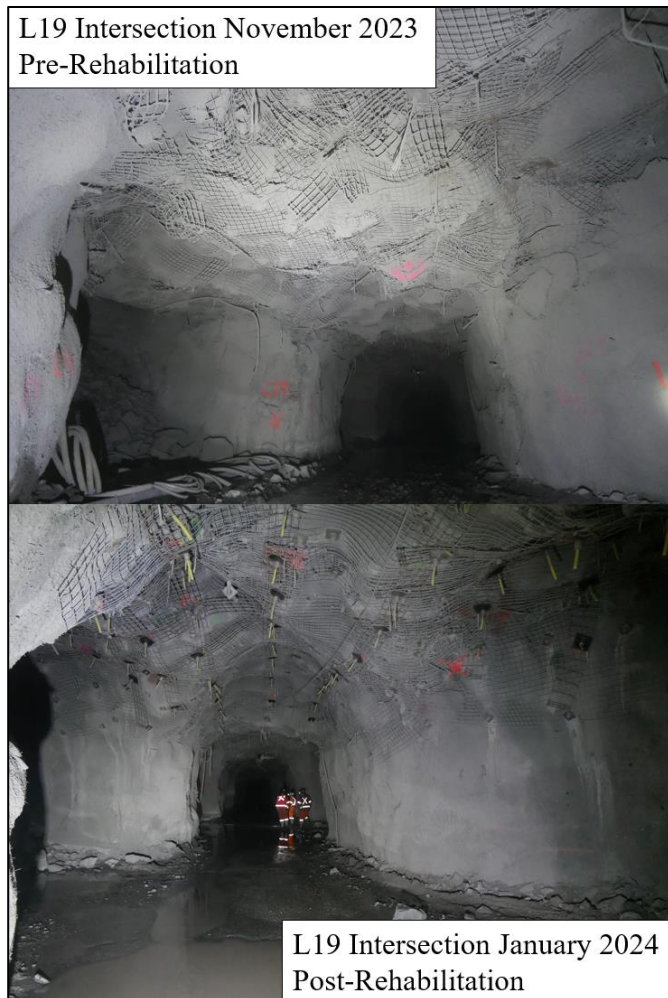
Figure 13. Pre and post rehabilitation comparison of L19 intersection rehabilitation. Both photos looking east towards EAC-7.
