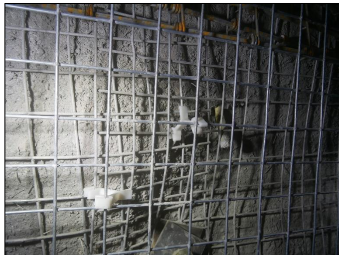
Figure 14. Plastic spacers used to hold a sheet of mesh in place to be sprayed over.
